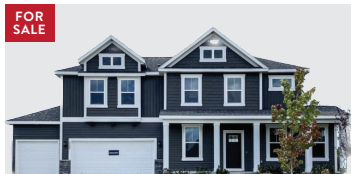
13 | BOSGRAAF HOMES 3237 ROCAWAY DRIVE HUDSONVILLE 49426
